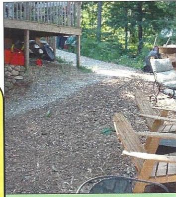
**Mulch**—Place mulch such as P&K Gravel's "fine erosion control mix" on bare soil.
